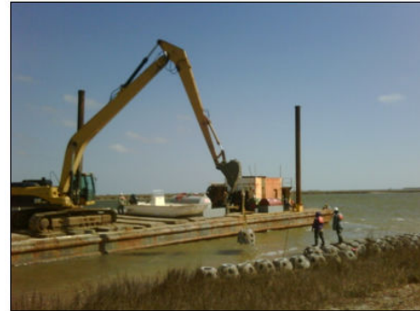
Bank Erosion Protection at Chocolate Bayou
